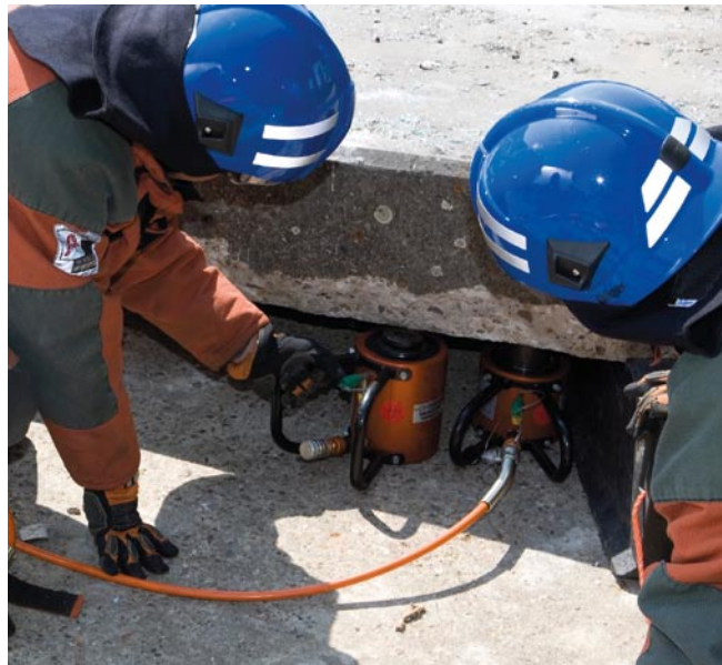
Two proportionally sized lifting jacks are used for heavy lifting
