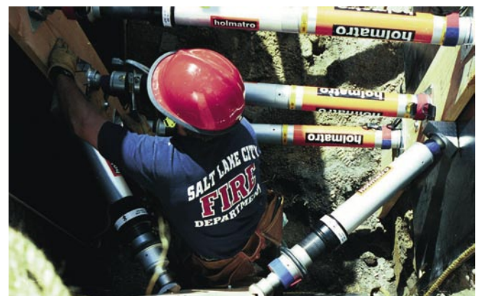
In a trench rescue, rescuers must create a safe working area around the victim from where rescue and emergency medical care can be performed
